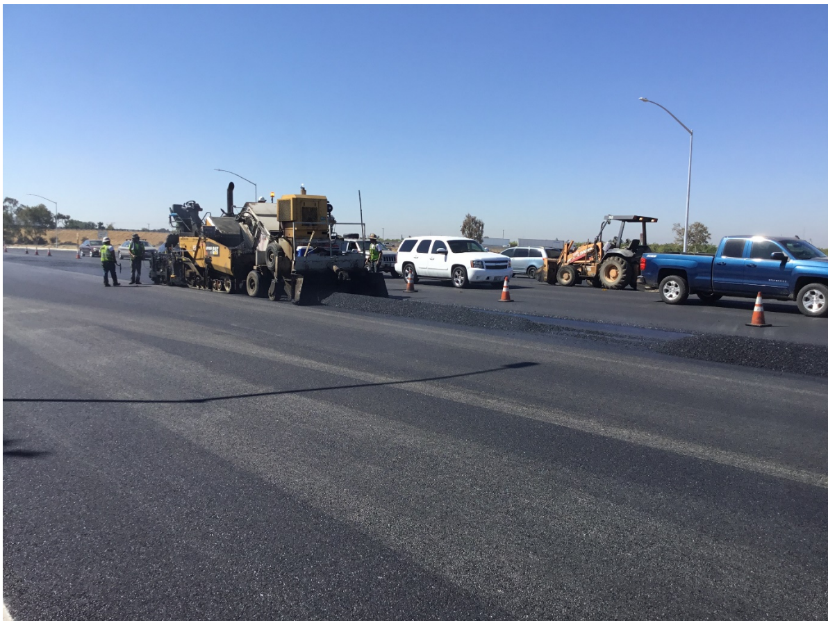
Placing Final Lift of Hot-Mix Asphalt
