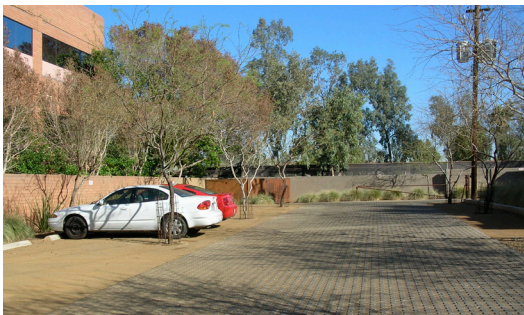
Low impact development standards, such as bioswales and permeable surfaces, help absorb rainwater to complement the stormwater drainage system and reduce runoff.
