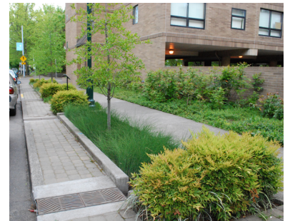
Bioswale within sidewalk.
